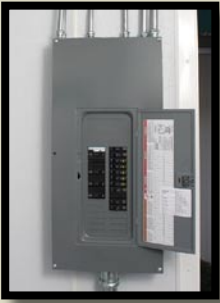
Load Center The SYNERGY unit is pre-wired and includes a 100 amp load center.
